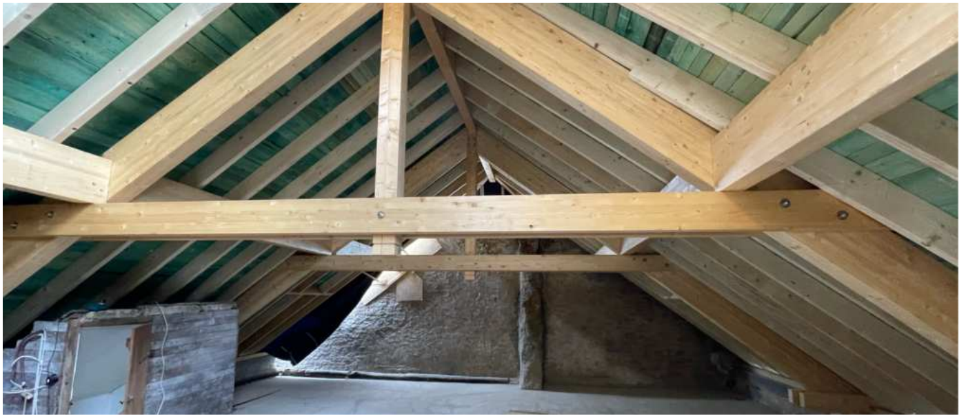
Roof framing and timber structures
